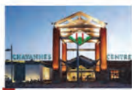
18 Chavannes Centre, Chavannes-de-Bogis (VD)
