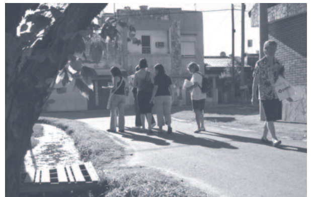
The GICP WSA team notes the lack of proper drainage along Juan Jose Paso Street.
