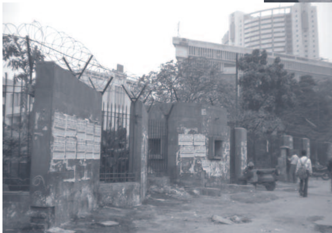
Boundary of a co-ed college near the main gate entry. Men frequently urinate in the area.
