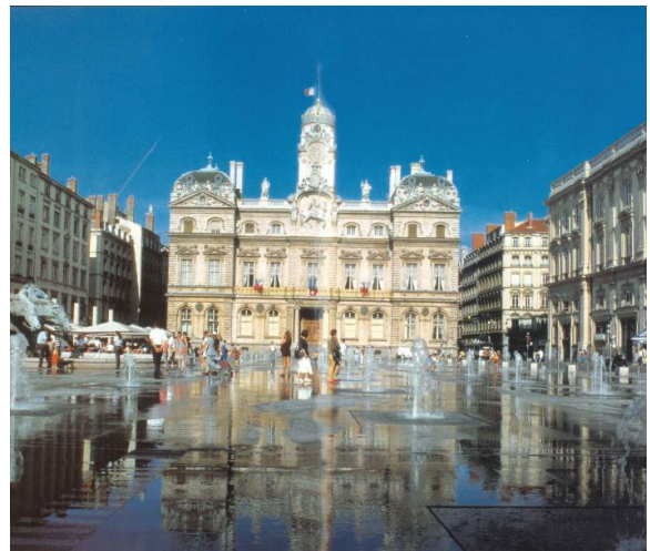
The new Place des Terreaux with underground parking structure
